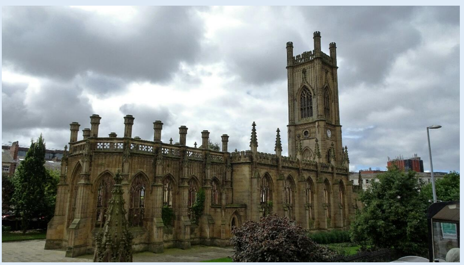
Bombed St Luke's Church
